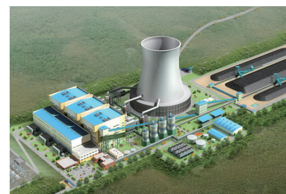
Tufanbeyli CFB Power Plant (450MW)
