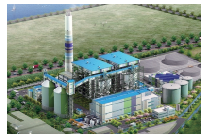
Yeosu CFB Power Plant(350 T/h CFBC BOILER)
